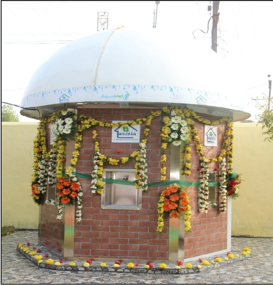
RO Water Plant at District Court premises, Karimnagar
